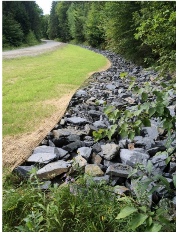
AFTER – Ditch was properly sloped and rock-lined to slow water velocity and five feet of the road shoulder was vegetated, leaving trees undisturbed.
