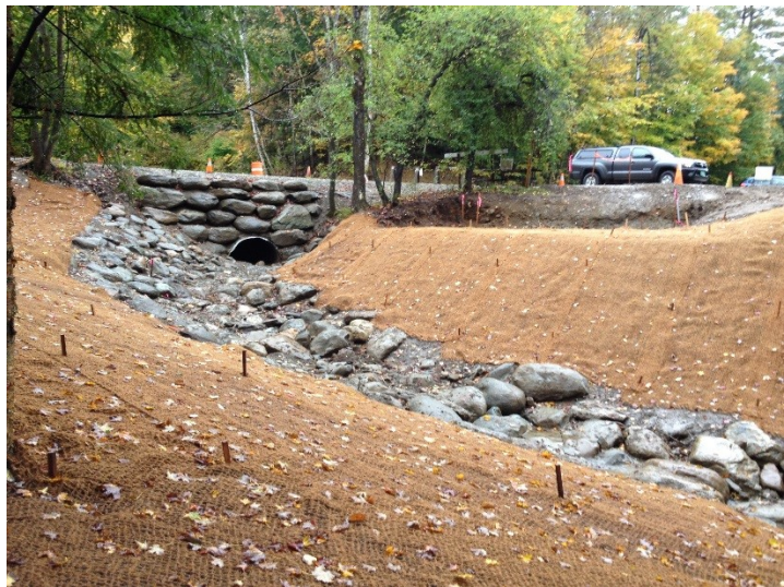
AFTER – Restoration work installed summer 2015 downstream of the town culvert at the head of the restored stream. The area will be planted in spring 2016.
