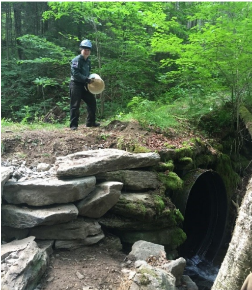
VYCC crew member deposits backfill into a newly constructed culvert wingwall.
