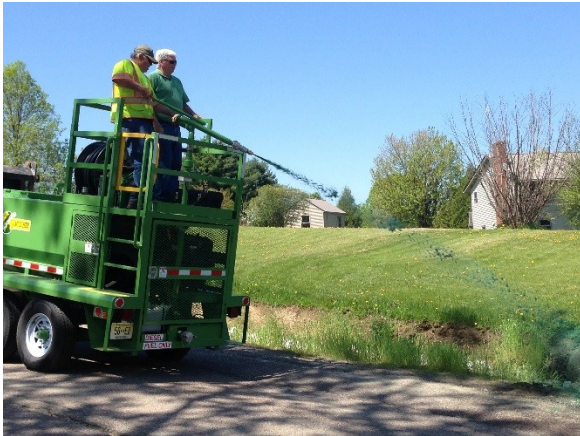
Hydroseeder equipment in use to quickly plant grass in a roadside ditch.
