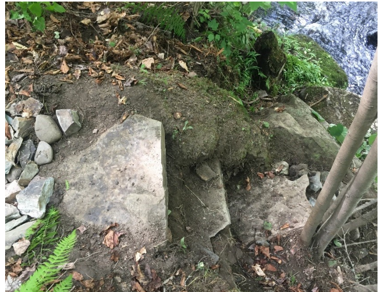
Energy dissipaters installed at the end of an armored drainage ditch.
