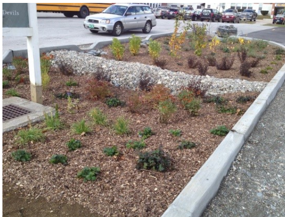
AFTER – Three bioretention/rain garden areas installed to treat stormwater runoff (above and below).
