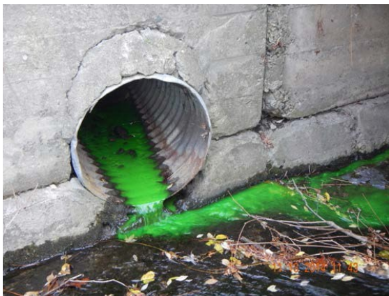
Dye indicative of raw sewage in stormwater outfall. This illicit discharge has been corrected since this photo was taken.
