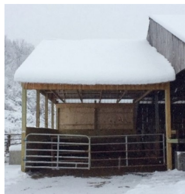
AFTER – Manure handling area with roof and containment wall installed to prevent polluted runoff.
