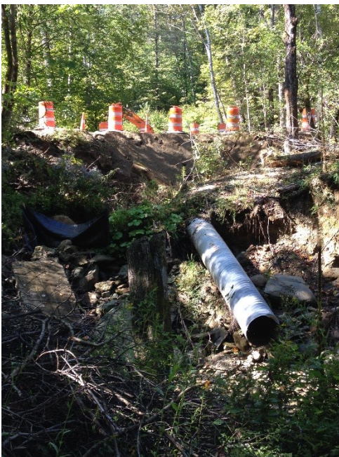
BEFORE – Damage after the 2013 flood downstream of the town culvert at the head of the gully.
