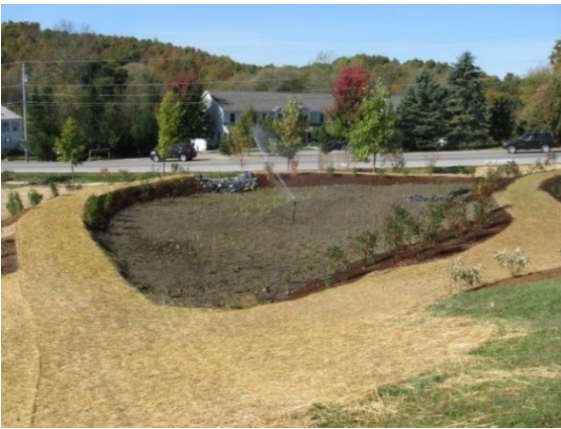
Rain garden consisted of two treatment cells designed to capture runoff before entering into the LaPlatte River.
