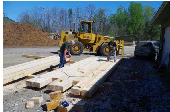
Bridge under construction at a May 2015 Portable Skidder Bridge Workshop to educate loggers on the how and why to use portable skidder bridges. Photo courtesy of the Winooski Natural Resources Conservation District.
