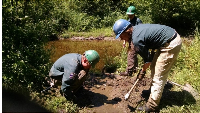
VYCC crews dig drainage ditches to allow standing water to drain from the roadway.
