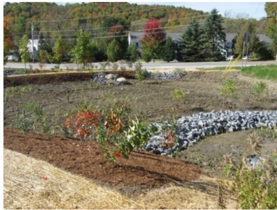
Rain garden consisted of two treatment cells designed to capture runoff before entering into the LaPlatte River.
