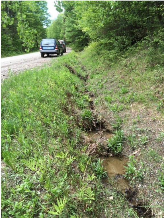
BEFORE – An eroded ditch on Kew Vasseur Road in Waitsfield sending sediment towards a nearby stream.
