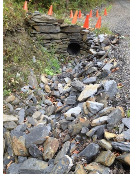
RIGHT – Stone culvert header to protect the soils around the culvert from eroding.
