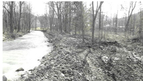
AFTER – The bank of White Creek after berm removal.
