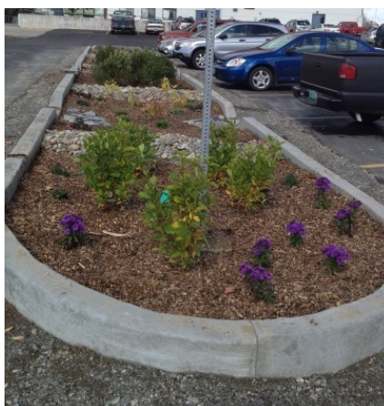
AFTER – Three bioretention/rain garden areas installed to treat stormwater runoff (above and below).
